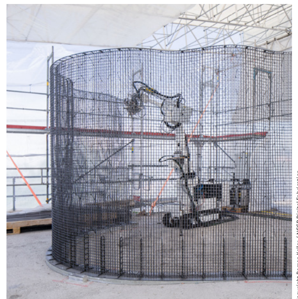
Copyright Roman Keller / NCCR Digital Fabrication
