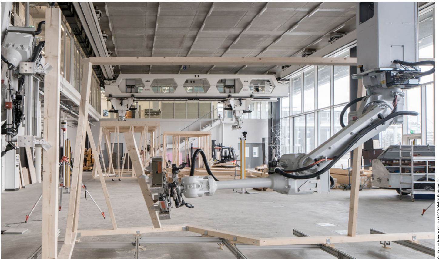
Copyright Roman Keller / NCCR Digital Fabrication
