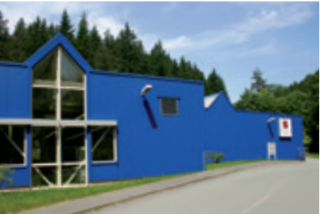
Werk 2 – Mellenbach Elektronikfertigung Facility 2 – Mellenbach Electronic Power Supplies Production
