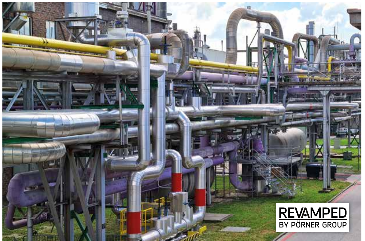
Following the final study from 2015/2016 and the execution phase starting in 2018, both revamp projects were completed in time.
