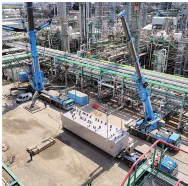
Everything according to plan and with precision: The new coldbox is lifted into place.
