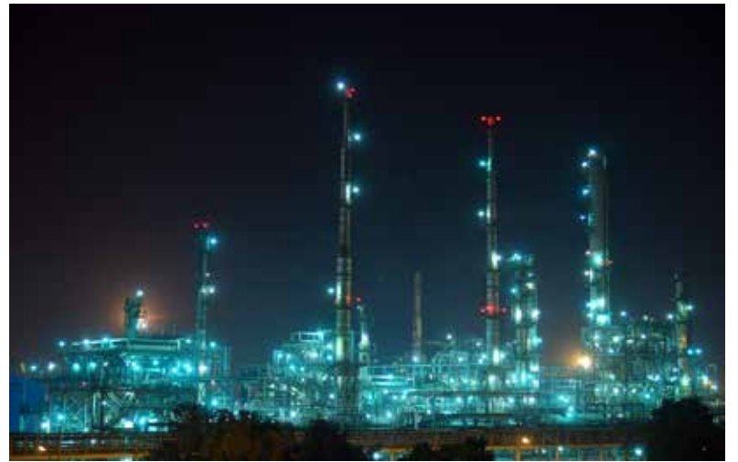
The Indian Oil refinery in Barauni will be expanded by a second Biturox® plant.
