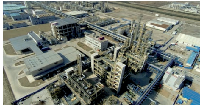
Evonik New fine chemical facility China Engineering, Procurement and Construction Management (EPCM). Gross floor area of the facility is 14,400 m 2 , the project consists of betaine, amido amines, ester, alkoxylation and quat production.
