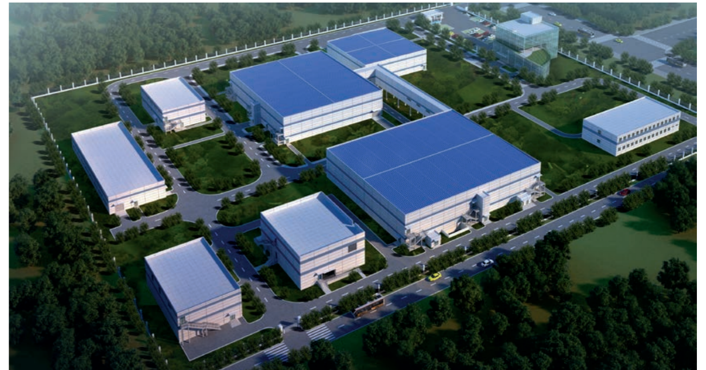
Merial Animal vaccine facility China Greenfield master planned facility implemented in phases to transfer operations from existing facility. New site includes animal building, QC laboratory building, production building, fill & finishing facility (vials), warehouse, utilities, WWT and office/cafeteria building.
