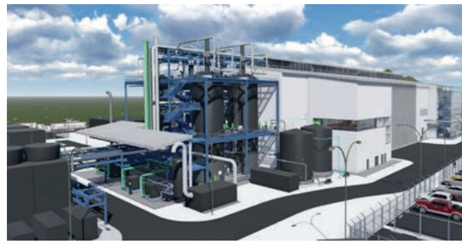
Verdezyne Inc. USA Design of a new greenfield Dodecanedioic Acid (DDDA) plant Malaysia Front end engineering design of a new greenfield facility to build the world's 1 st bio-based crude dodecanedioic acid (DDDA) plant with production capacity of 6,100 tons/annum of diacids.
