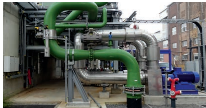
BASF High purity nitric acid plant Germany Exyte as EPC provider and responsible for technology integration. Two million plus safe man hours.
