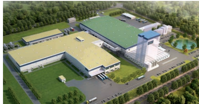
Kerry New food flavors plant and distribution center China EPC and GC for a food flavors and ingredients production facility which is adjacent to the existing production facility including a recently completed distribution center.
