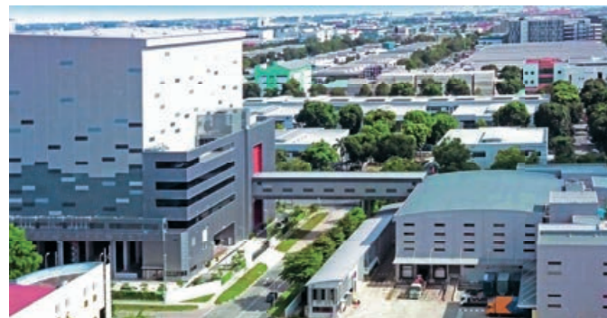
Coca-Cola (Pacific Refreshments) New automated warehouse and link bridge Singapore The 6,000 m 2 four-story concentrate plant with overhead bridge having a dual two-way fully automated conveyance system transports the finished products from the manufacturing facility to the storage.
