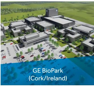
**Bio-Pharma Campus 42,000m<sup>2</sup>:** EPC project, incorporating four independent prefabricated modular SUT MAB production units (each 2,500 m<sup>2</sup>).
