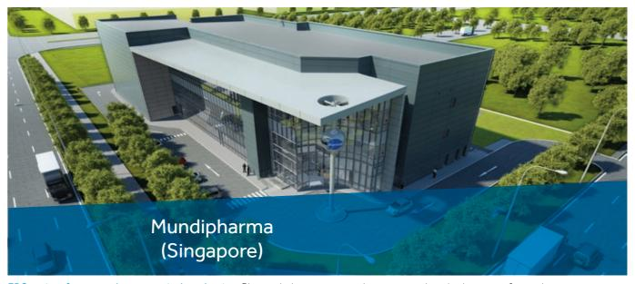
**EPC project for a new pharmaceutical production:** Plant including a 3-storey pharmaceutical grade cleanroom for single use technology. Designed for further expansion to significantly increase production capacity of antiseptic products in future.
