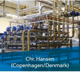
Capacity expansion of starter cultures production: EPC, utilities, solid handling, FM mixer, mixing tanks, UHT, large scale fermenter, homogenizer, cryogenic tank, CIP, eluate, tie-ins to existing plant.
