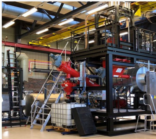
1 MW pilot plant with the Torrgas / TAF / DBI process for the production of synthesis gas from torrefied waste wood in Delfzijl / The Netherlands; a 25 MW plant is planned
