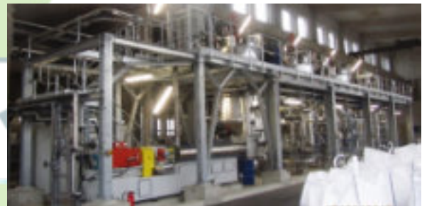
Engineering and construction of a plant for the production of 4,000 TPA fully synthetic waxes from polyethylene and polypropylene through depolymerization; Webau / Germany, 2016
