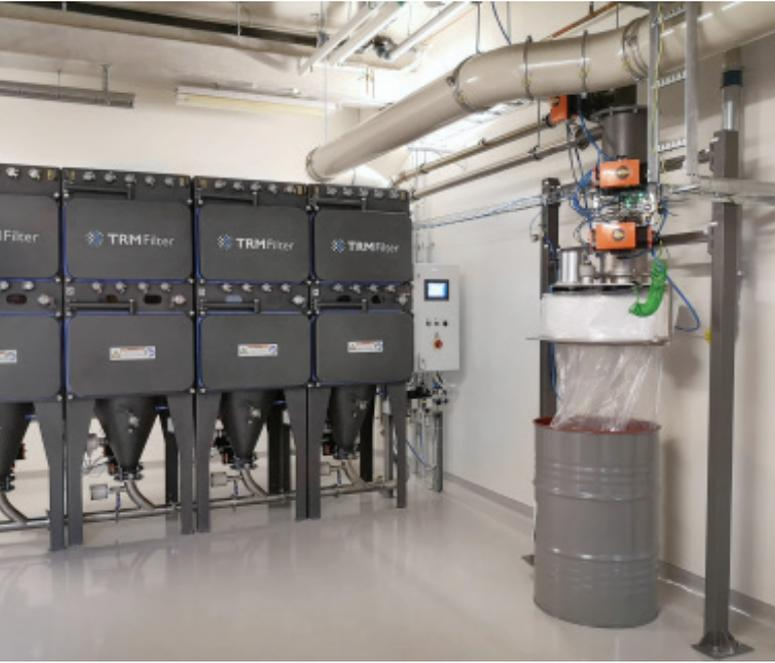
Dedusting filter system type ECR by TRM Filter with central dust collection and continuous liner in pharmaceutical application.
