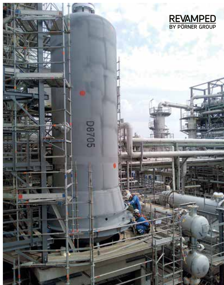
Thanks to good engineering, the 55-ton reactor fits perfectly on the foundation. All equipment was replaced without a hitch.
