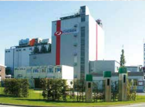
Plant for the production of 15,000 t/a fuel and 2.3 MW electricity from 65,000 t/a wood, based on pyrolysis, gasification, synthesis gas purification and conditioning, Fischer-Tropsch synthesis, electricity and oxygen generation, built in 2007
