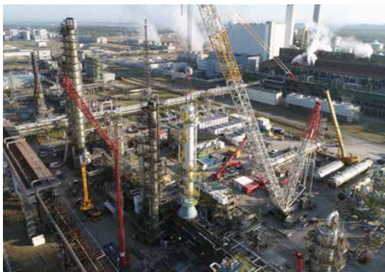
Lift of new extraction column under ideal conditions in April 2020
