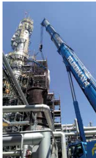
Lifting of the old reactor that reached the end of its life
