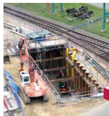
The tub to accommodate the larger EO tank is being prepared, sheet piling with groundwater lowering, excavation depth approx. 6.5 m.
