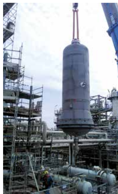
Installation of the new reactor on a weekend in June 2020
